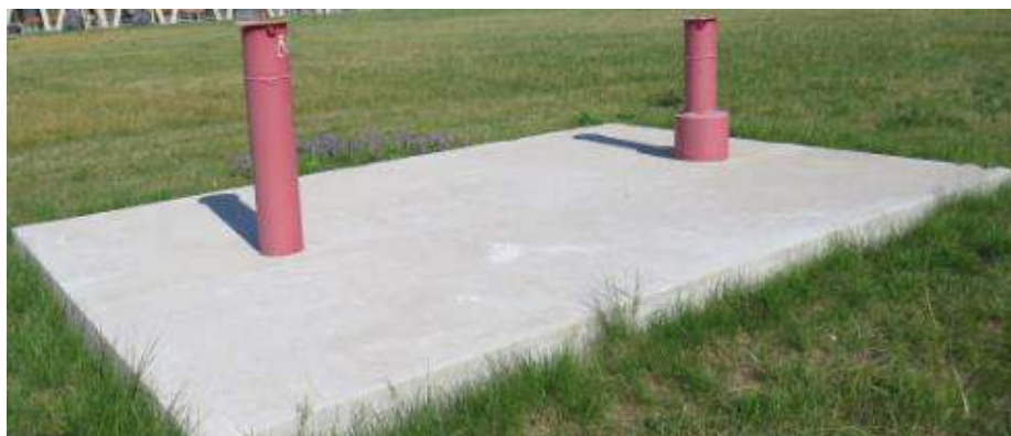
Figure 8.6 Piezometric well cluster
