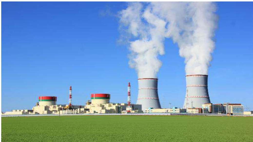
Figure 2.1 – Belarusian Nuclear Power Plant
