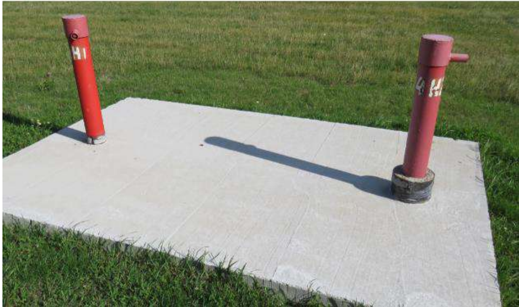
Figure 8.6 - Piezometric well cluster
