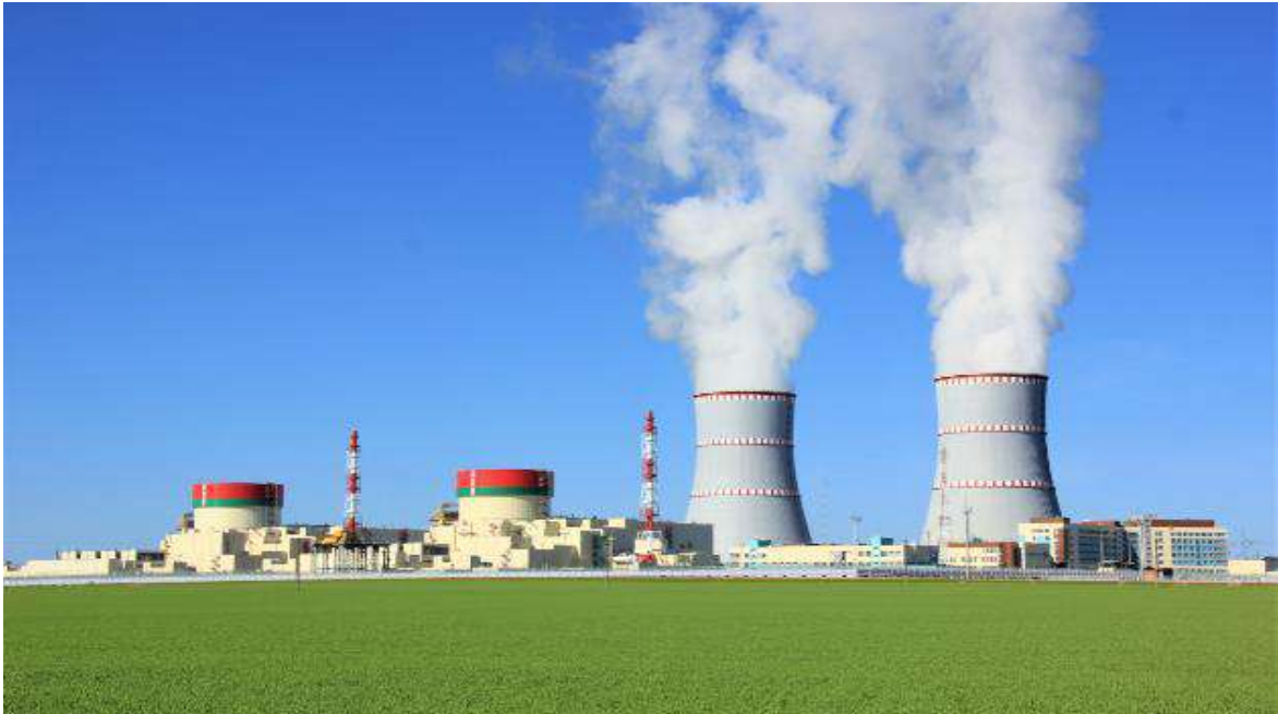
Figure 2.1 - Belarusian Nuclear Power Plant
